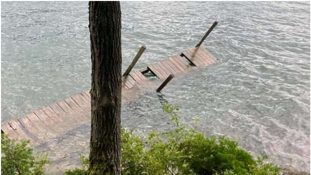
Boat wakes can cause damage to docks & moored boats
